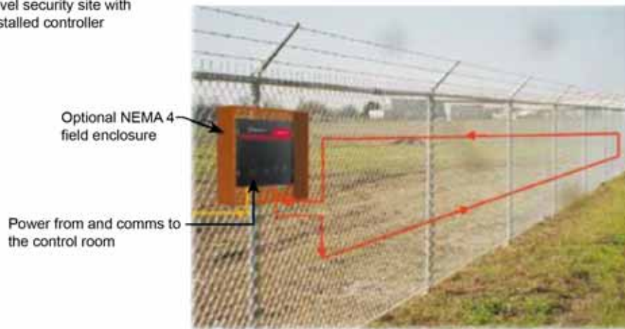
Figure 64 Fence-Mounted Controller as part of a PIDS
