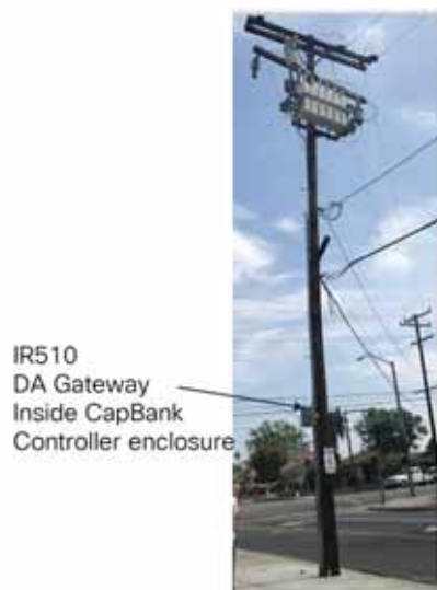
Figure 150 IR510 Overhead Line Installation
