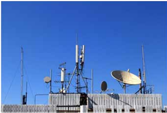
Figure 135 Co-Site Interference Example
