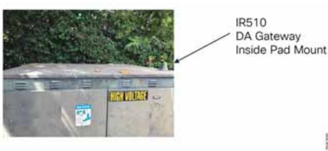
Figure 151 IR510 Underground Line Installation
