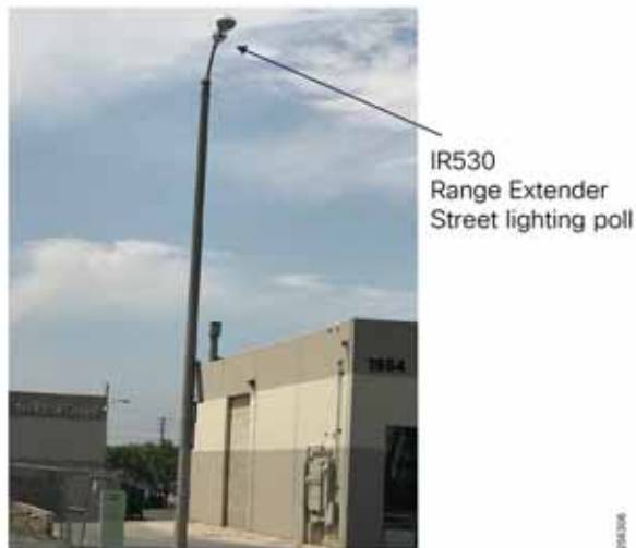
Figure 152 IR530 Street Lighting Poll Installation
