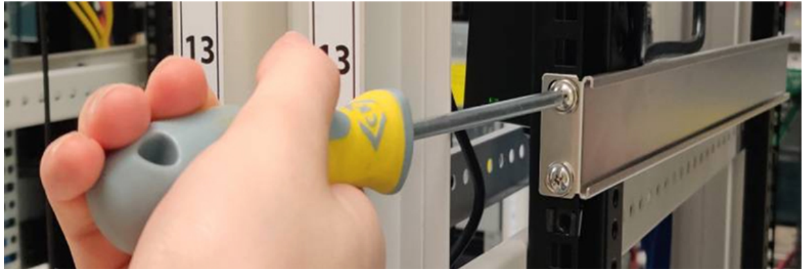
Figure 8: Attaching the left hand side rail.
