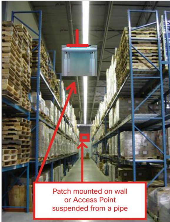
Figure 64. AP placement in a warehouse environment
